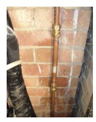
This is the Standard Vortex Water Revitalizer 1"which was installed in the Lambton Park Hotel. It was installed using compression fittings.
